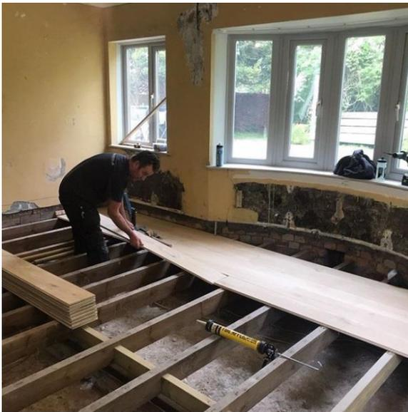
A nail down installation can be over any wooden subfloor.
