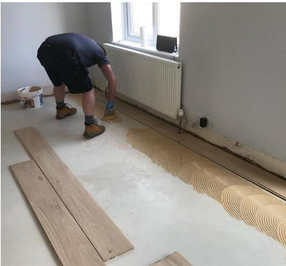
This method requires the floor to be free of dust, flat and even. The adhesive should be applied in accordance with the relevant MS polymer adhesive manufacturer's instructions.
