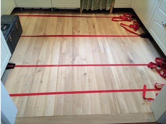
Tap against the tongue; tapping the groove may damage the edge.
