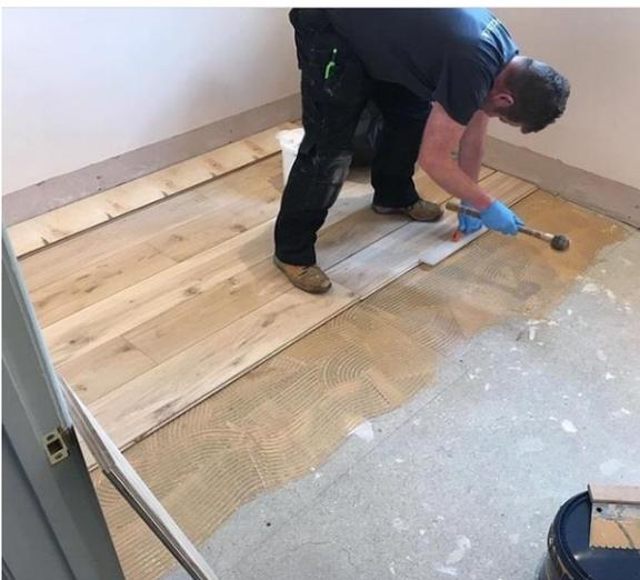
Spread the MS Polymer [adhesive](#) using a coarse notched trowel along the working line.
